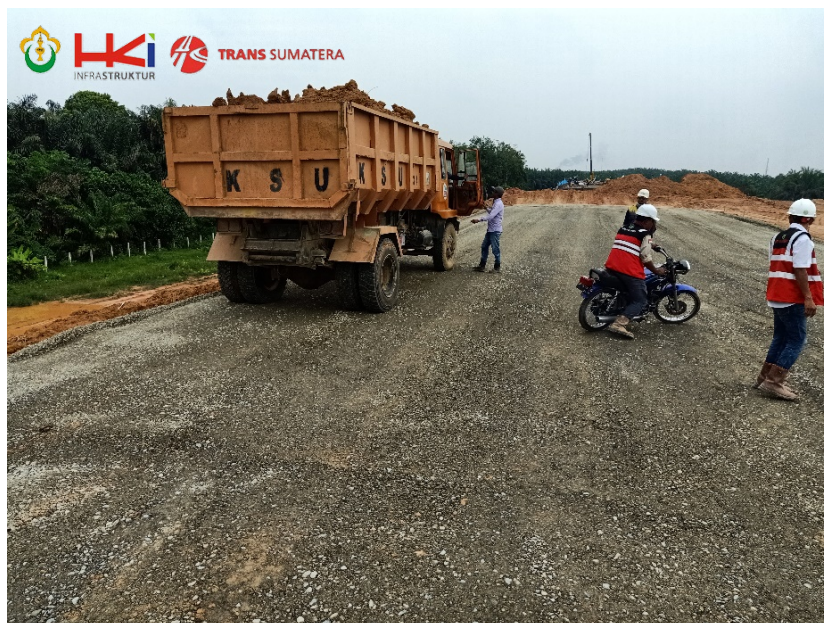
Gambar C.4 Profolling lapisan drainase
