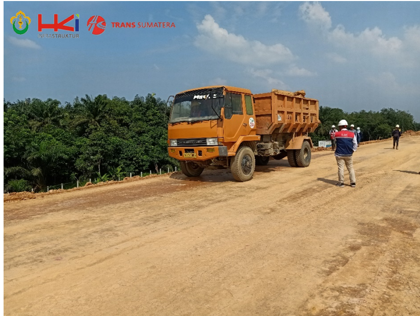
Gambar C.3 Profolling tanah timbunan
