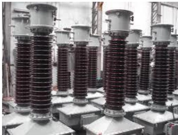
Gambar 2.13 Transformator arus
