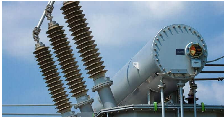
Gambar 2.10 Bushing Transformator
